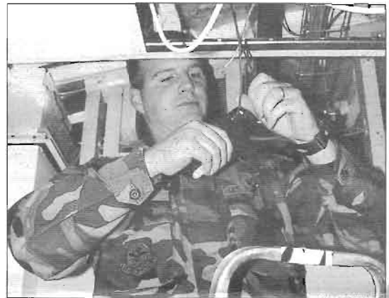
Senior Airman Paul Tobkin installs electrical service to an office.
