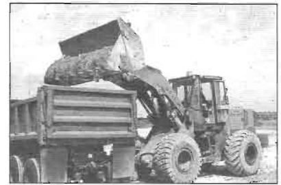
Wing civil engineers moved dirt for a runway construction project.
